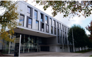
Office, Fraunhofer IWU, Dresden
