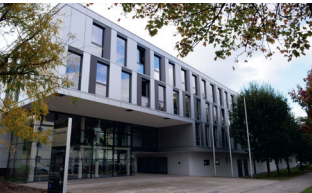
Office, Fraunhofer IWU, Dresden
