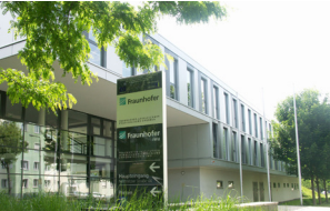
Office, Fraunhofer IWU, Dresden
