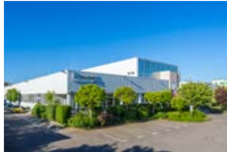
Main building of the IMM
