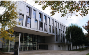
Office, Fraunhofer IWU, Dresden
